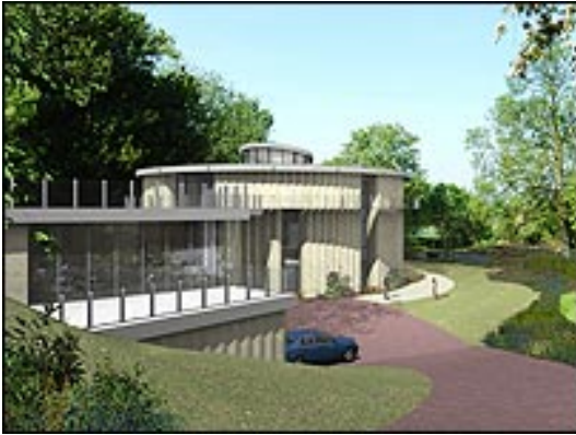
Figure 11. Solar-powered building that can rotate on wheels and tracks, invented by Hamilton, a British inventor (BBC Chinese, April 13, 2007. Retrieved January 30, 2009, from http://news.bbc.co.uk/1/hi/newsid_6550000/newsid_6554500/6554549.stm )
